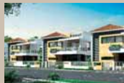
APARNA HILLPARK GARDENIA (Work in progress) 116 Premium Luxury Villas, Miyapur, Chandanagar
