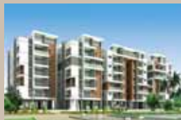
APARNA KANOPY TULIP (Work in progress) 360 Value apartments - Phase 1A Gundlupochampally, Kompally
